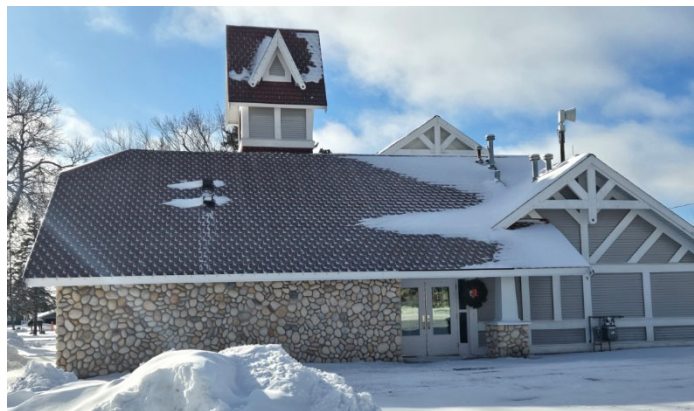
Photo showing building entrance at north side to parking lot.
