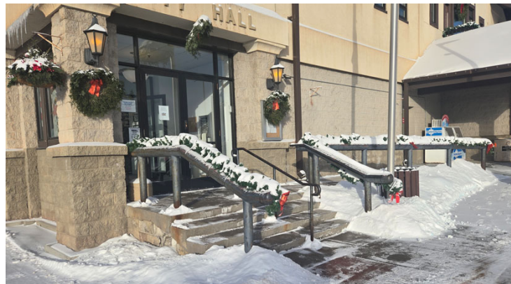
Photo showing the sloped ramp, with rails, leading to the main entrance of city hall.
