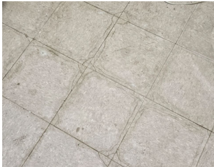
Photo showing typical condition of VCT flooring within office area.
