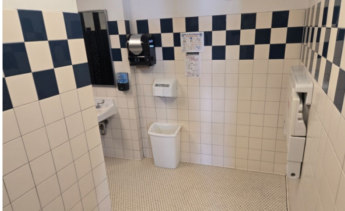
Photo shows typical interior finishes at restrooms.
