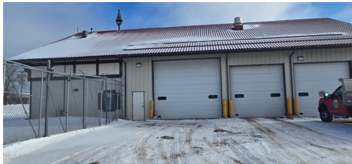
Photo showing west façade at employee entrance and equipment bay entry.
