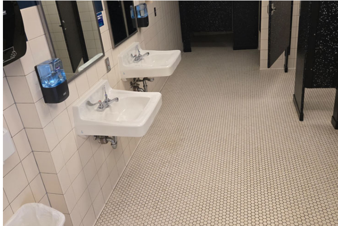
Photo shows wall mounted lavatory with open knee space.
