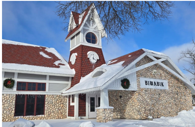
Photo showing building entrance at east side to street.
