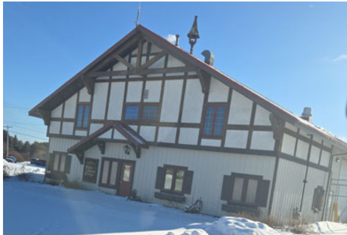
Photo of north façade of building facing public parking lot.
