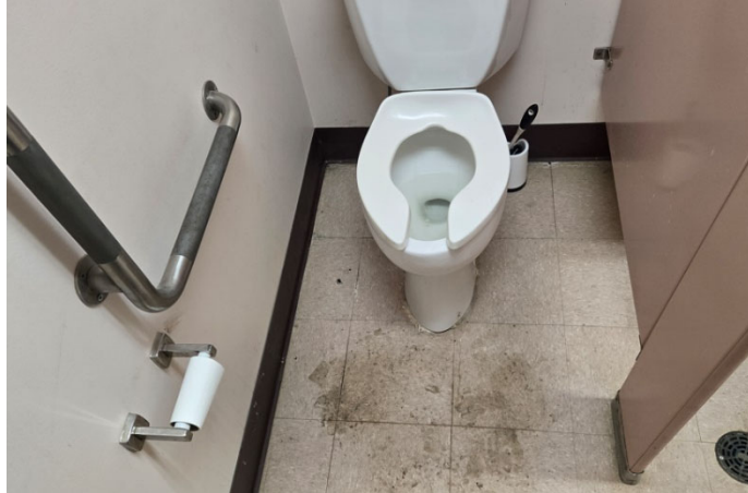
Photo showing typical restroom stall configuration.
