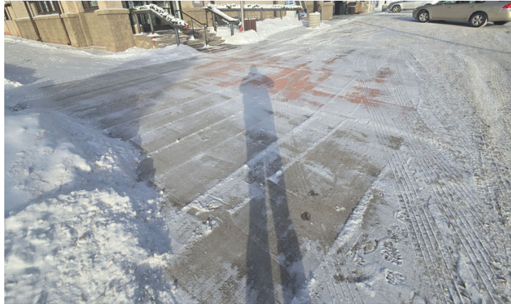
New concrete walk along street and into parking lot area.
