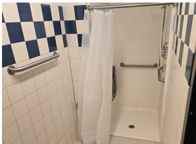
Photo shows typical accessible shower stall room.
