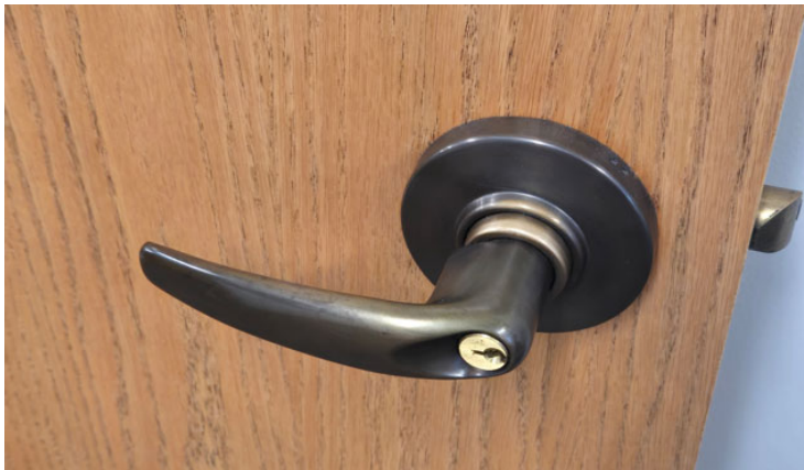
Photo showing graspable door lever handle.
