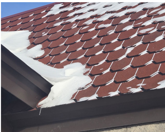
Photo of asphalt shingles.
