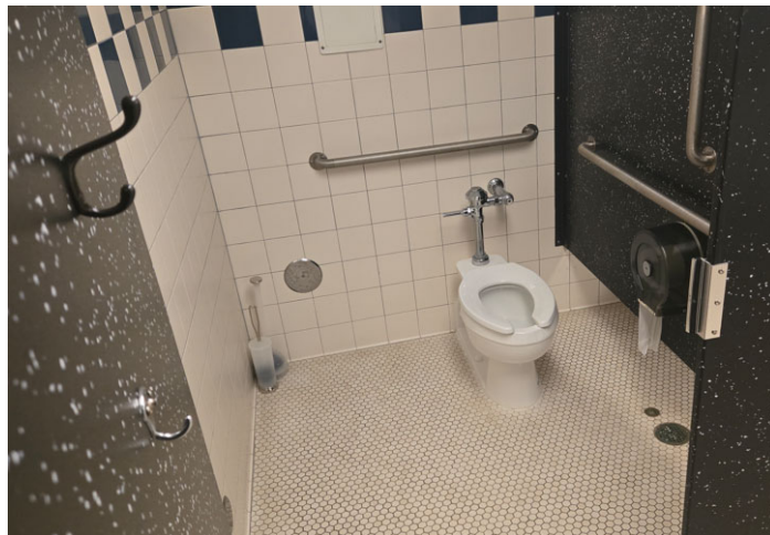
Photo shows typical accessible toilet stall within partition.
