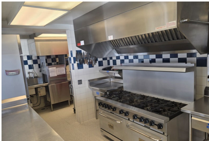
Photo shows typical finishes at commercial kitchen.
